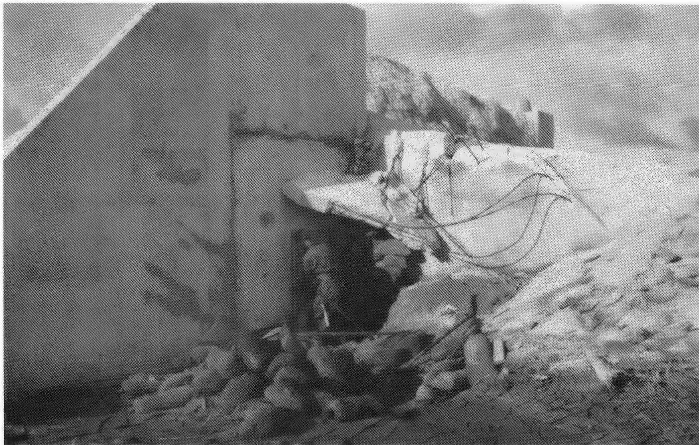
FIGURE 5-35. IVY MIKE POST-SHOT STATION 520 ON RUCHI ISLAND; JOHN MALIK ON REENTRY ON D + 4 (5 NOVEMBER 1952); DOSE RATE OF 3000 R/HR AT 1 HR HAD DECREASED TO ABOUT 12 R/HR. (30)
